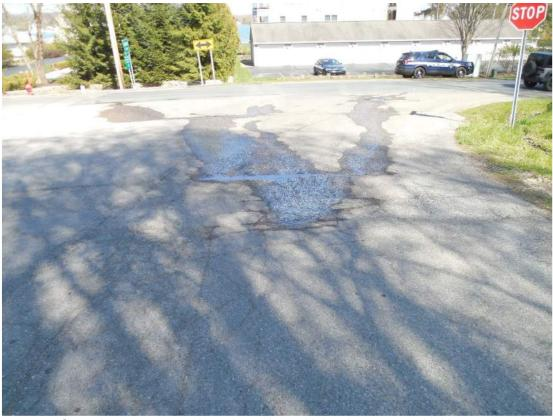
Groundwater seepage through cracks and joints in pavement looking east
