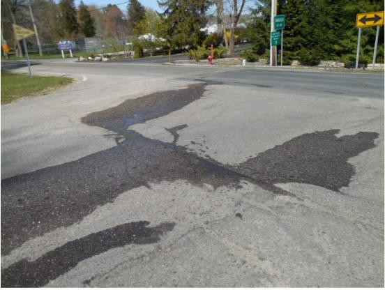
Groundwater seepage through cracks and joints in pavement
