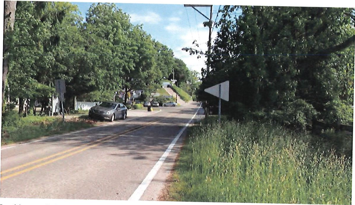
Looking north from the site
