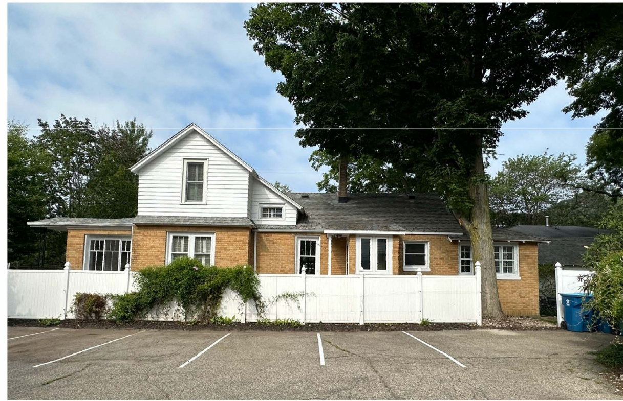
1 CONTEXT PHOTO - EXISTING EAST ELEV
