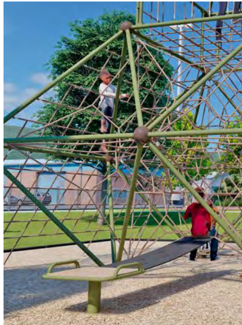
Transfer platform for net structure
