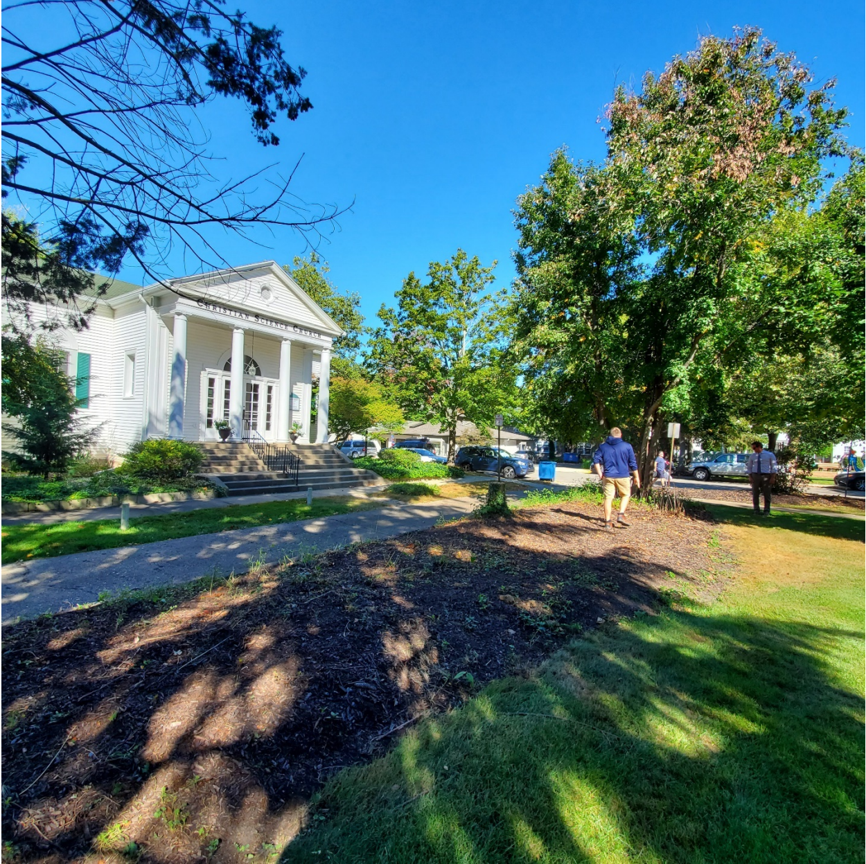
Figure 10: Mulch bed and tree removal along west side
