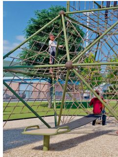
Transfer platform for net structure
