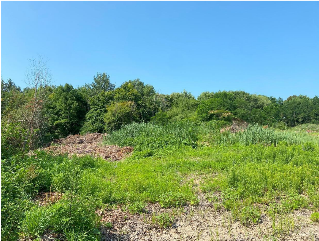
Figure 5: Photo of disturbed storage yard showing frequent soil disturbance and predominantly invasive and noxious plant species.
