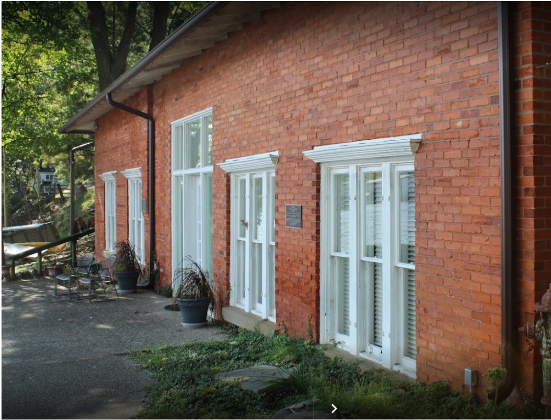
Existing Pumphouse Picture
