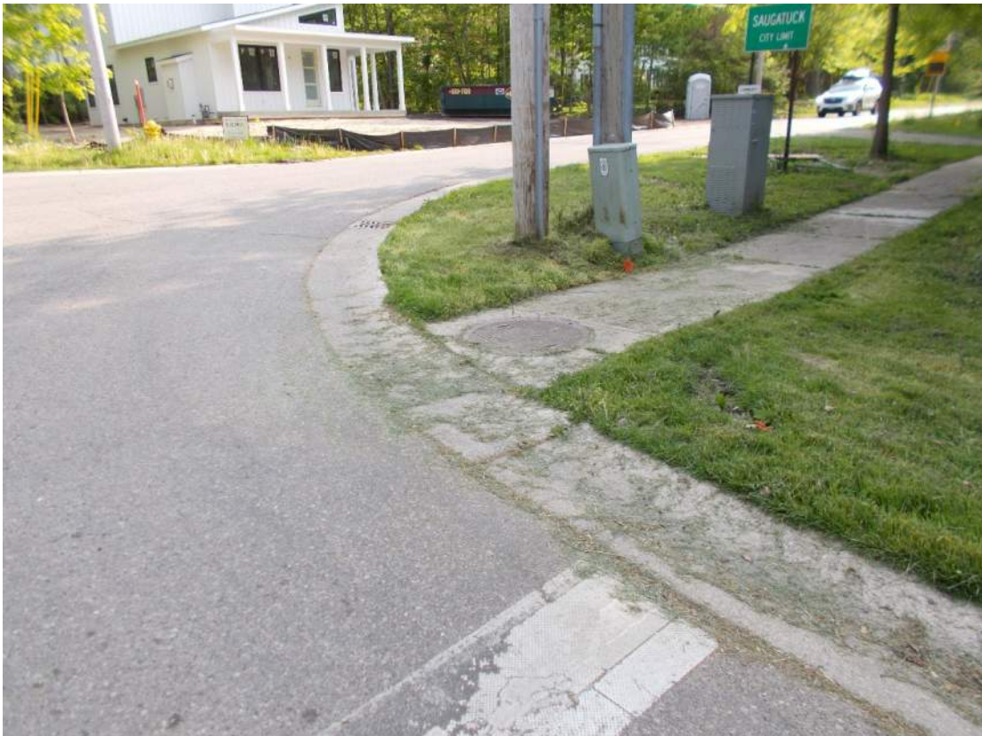
Sidewalk ramp in northwest quadrant of Maple Street and Allegan Street
