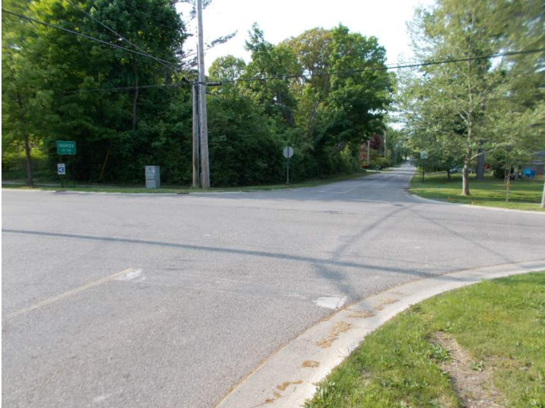
Maple Street at Allegan Street looking north
