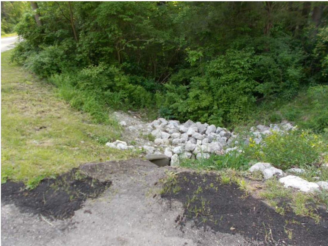
City stormwater outfall at Maple and Mason Street
