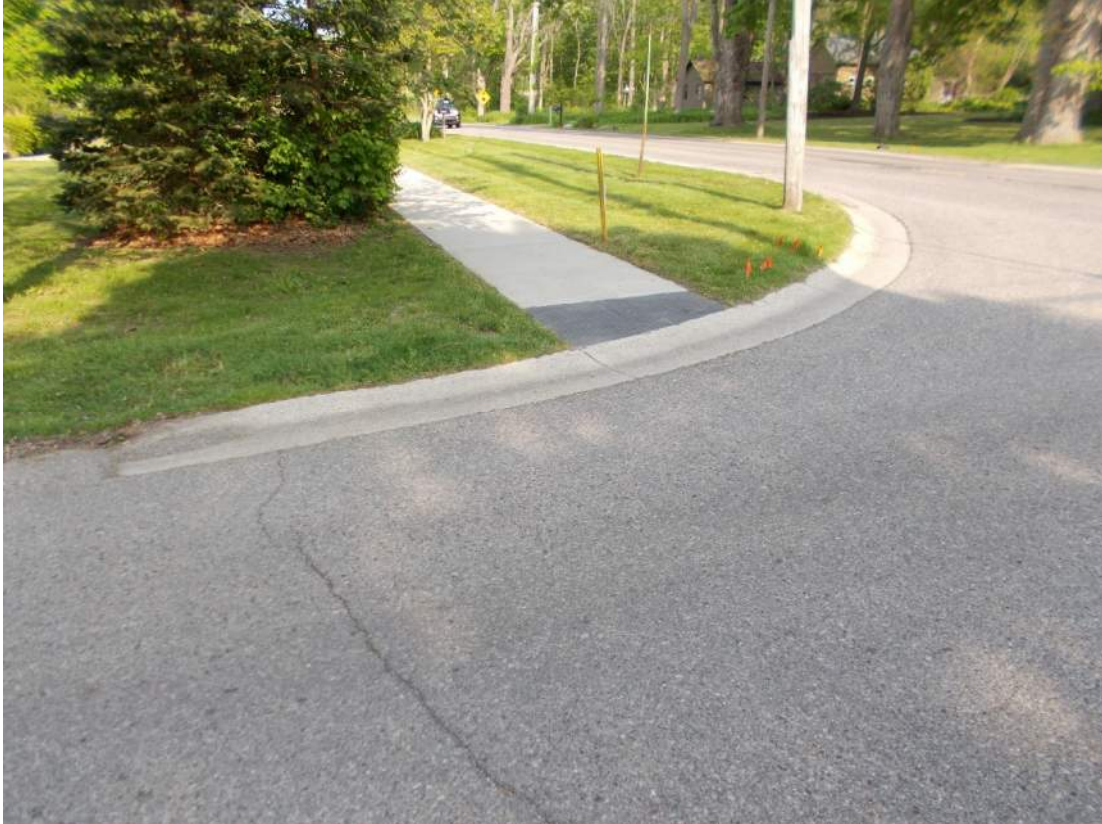
Sidewalk ramp at northeast quadrant of Maple Street at Allegan Street
