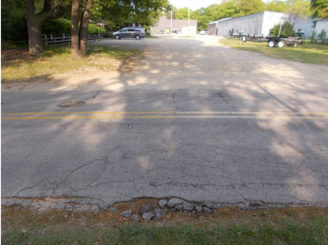
Saugatuck Township Fire District rear access on east side of Maple Street
