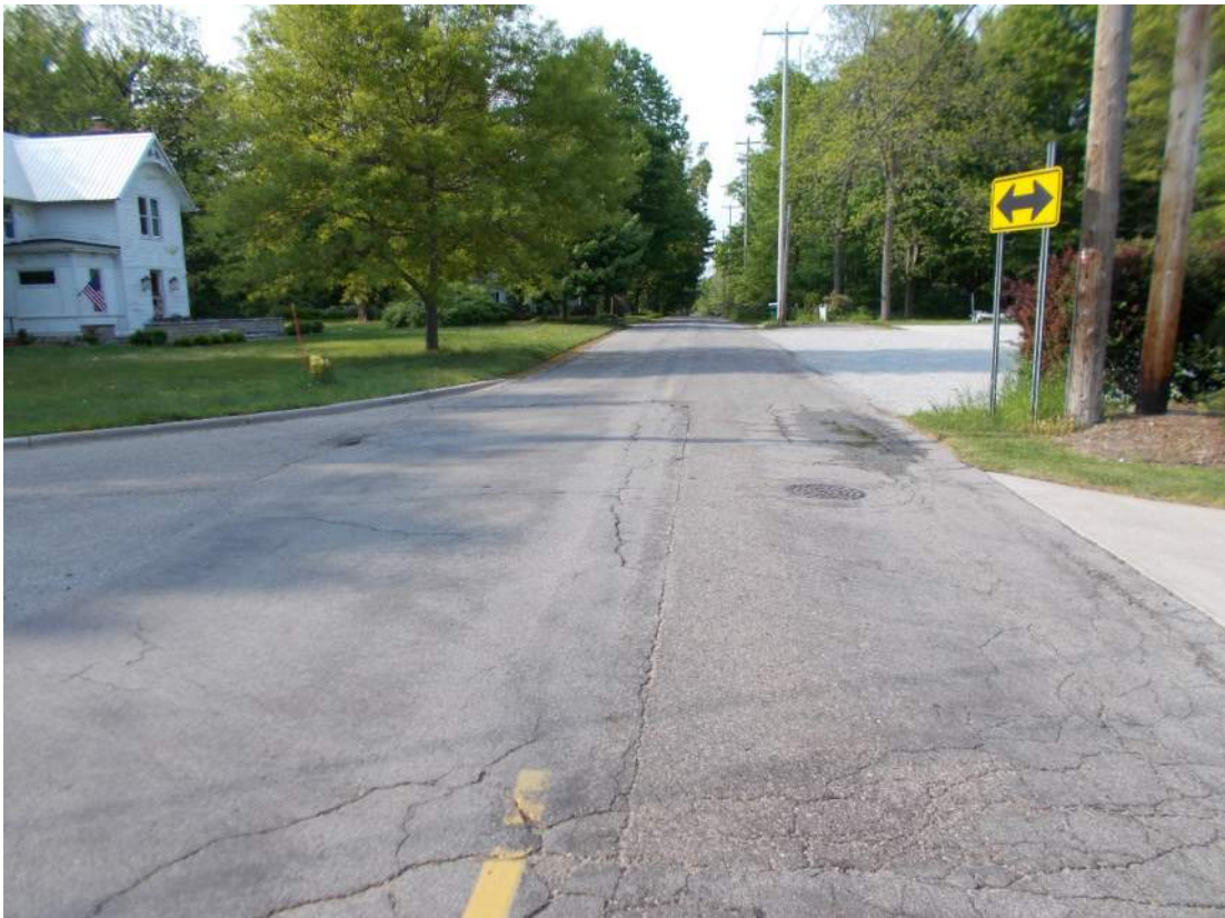
Maple Street at State Street looking north
