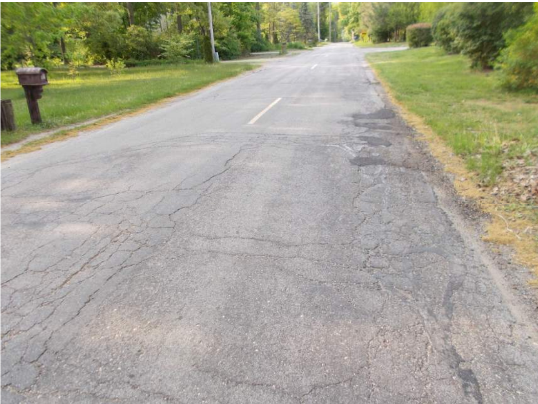
Maple Street north of Singapore Drive looking north
