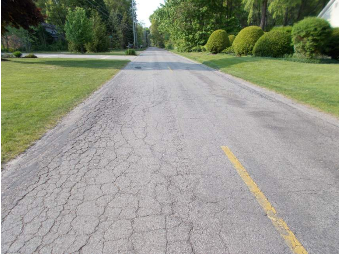
Maple Street south of Ridgeview Lane looking north
