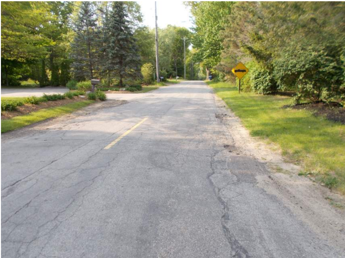
Maple Street looking north from Department of Public Works
