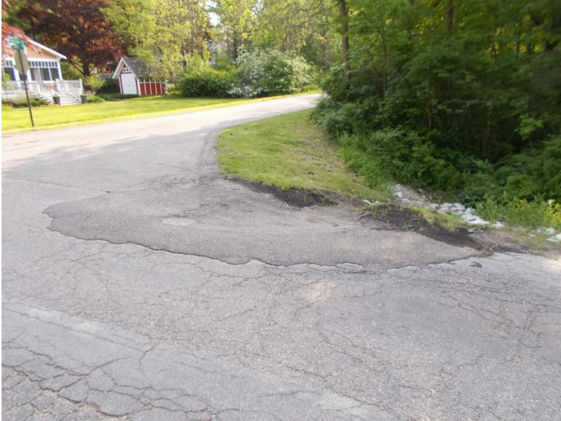
Spillway area in northwest quadrant of Maple Street and Mason Street
