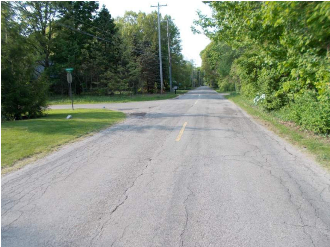
Maple Street looking north toward Ridgeview Lane
