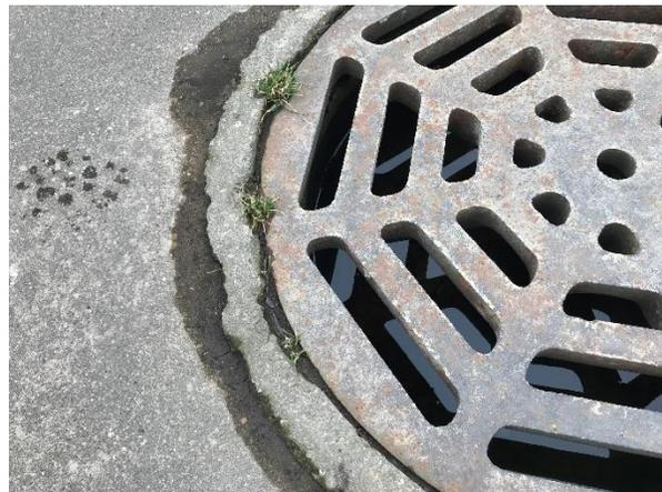
Figure 13 – Water level just below the frame
