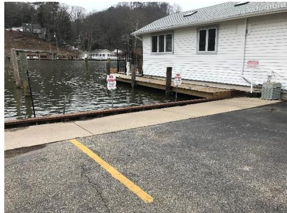
Figure 15 – Adjacent parking and sidewalk settlement
