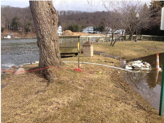
Figure 28 – Sandbags, sump pump and discharge
