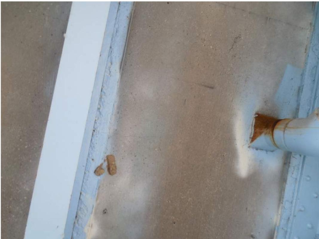
Cracking on bottom of deck near deck drain penetration
