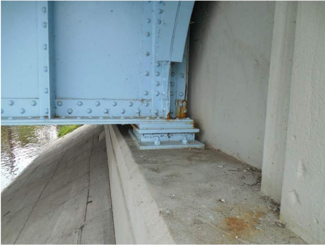
Paint failure with corrosion bleeding at bearing
