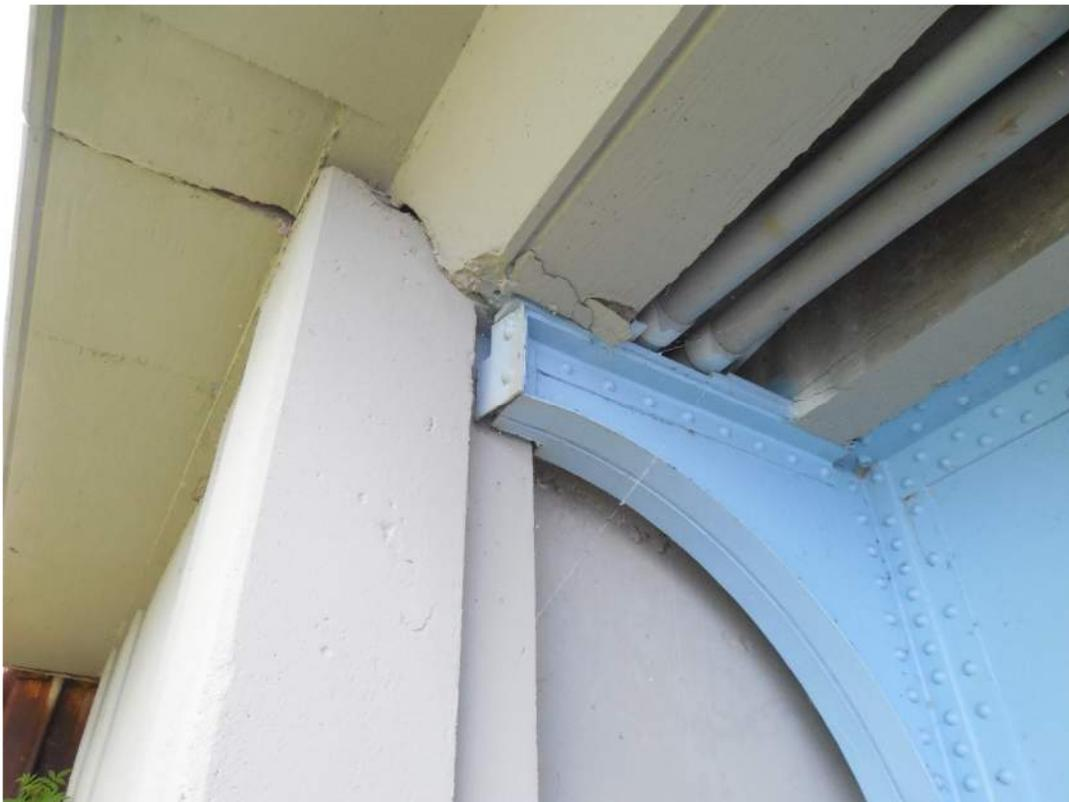
Concrete spalling at sidewalk support bracket
