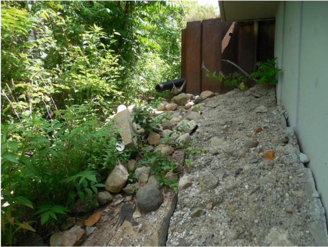
Underdrain outlet failure in northwest slope
