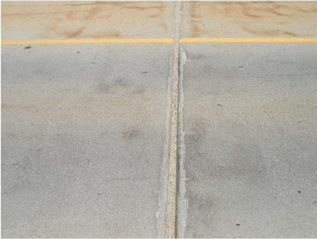
Debris in expansion joint and overlay raveling along the joint
