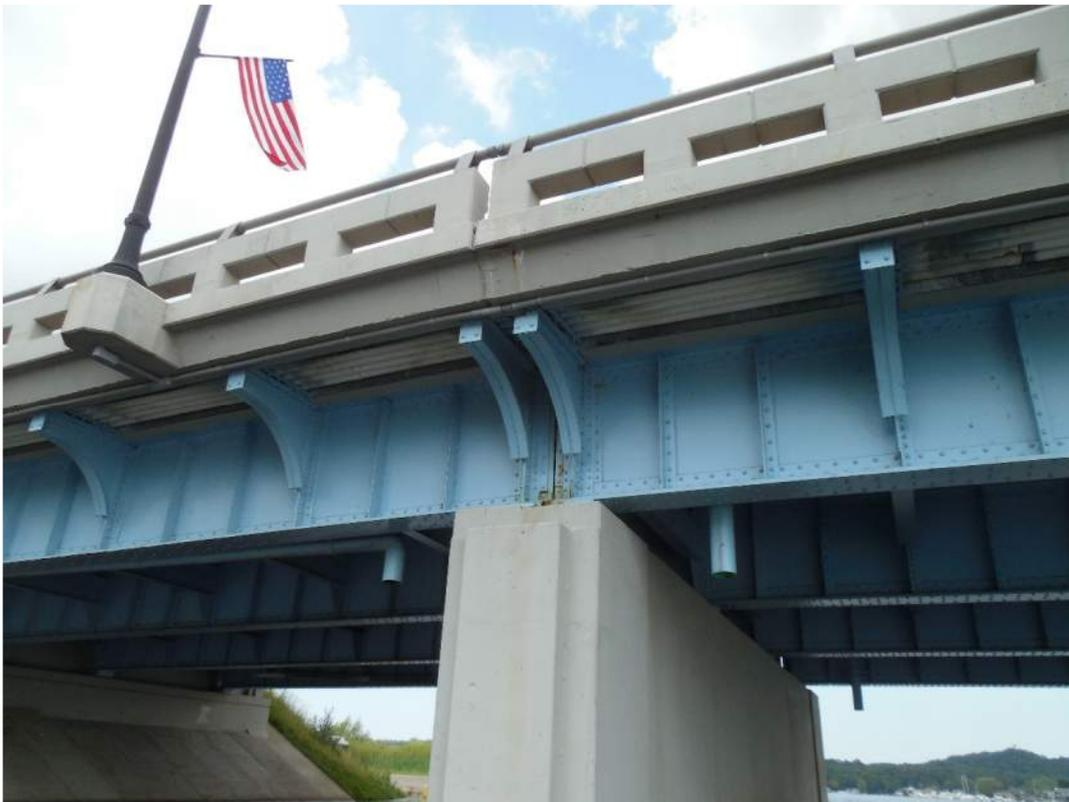
Paint failure and corrosion at pier
