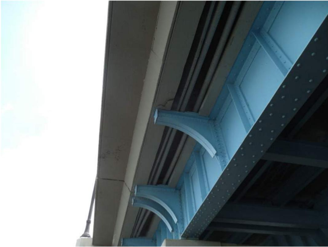
Concrete spalling at sidewalk support bracket
