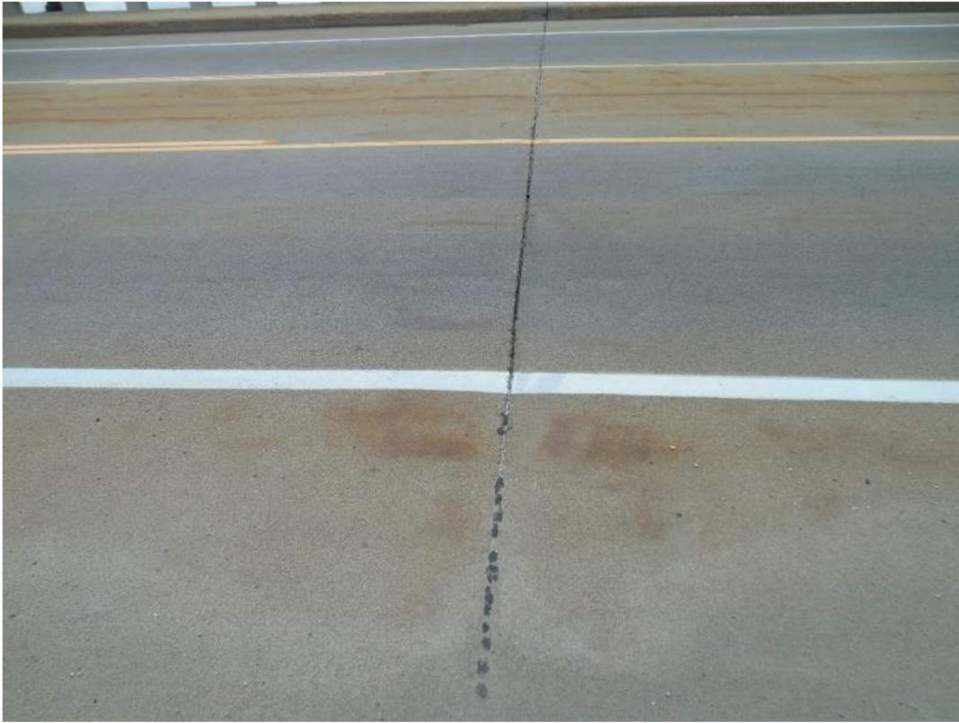
Deterioration of joint seal at fixed joint, pier 3
