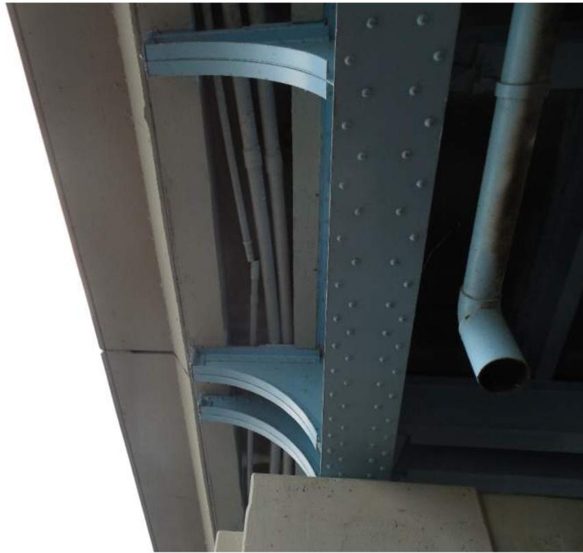
Joint separation in conduit beneath west sidewalk
