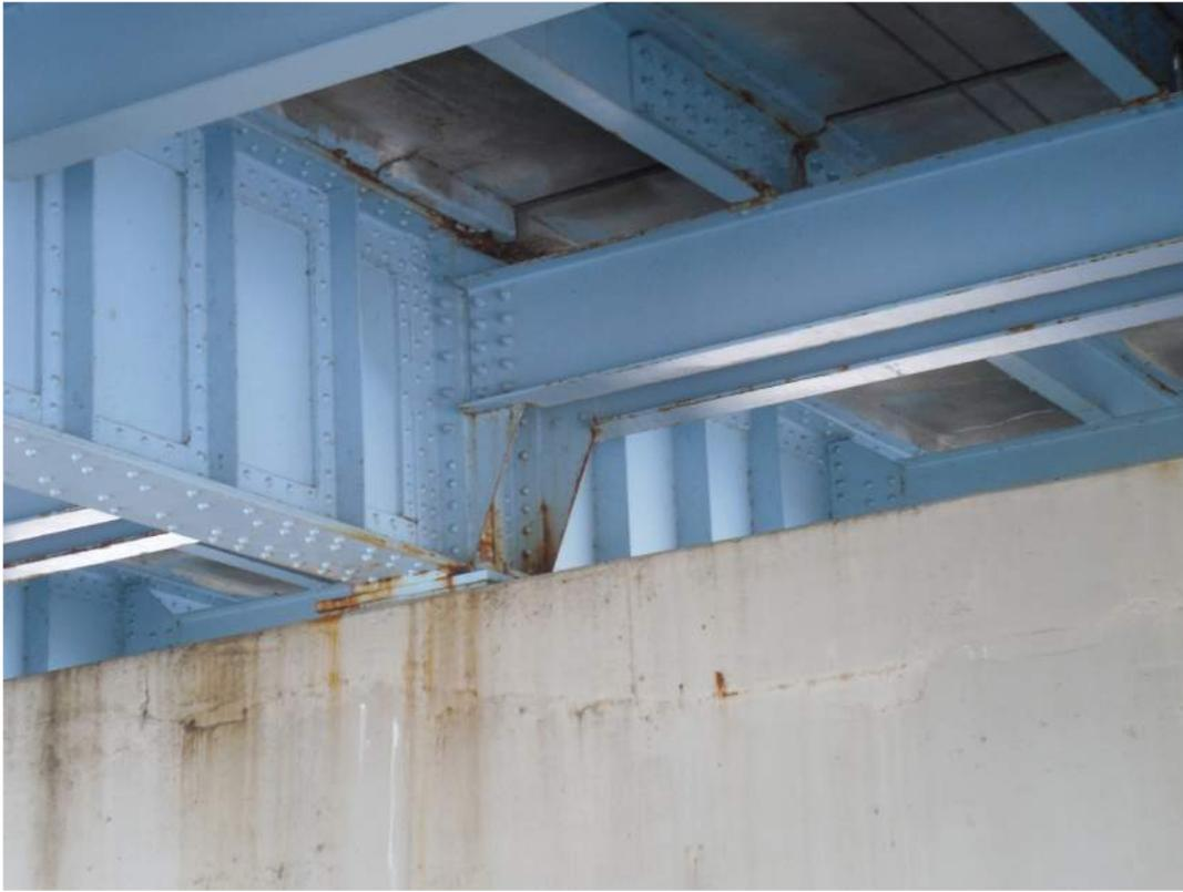
Paint failure with corrosion bleeding at pier
