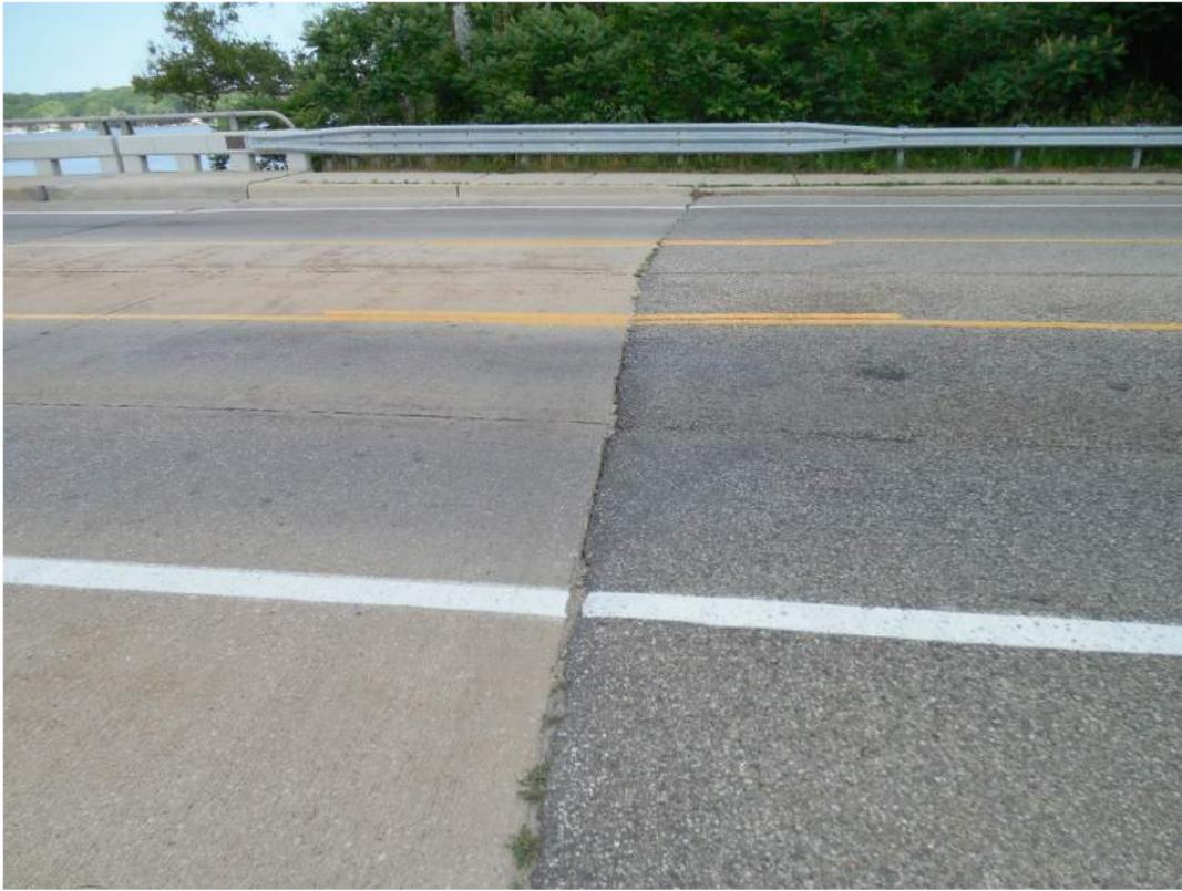
Joint separation along asphalt-concrete joint
