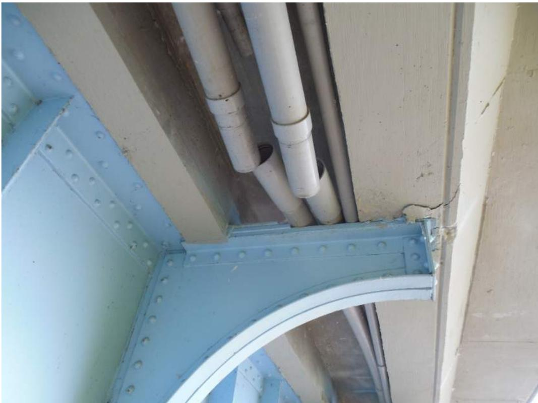
Separated expansion joints in conduit
