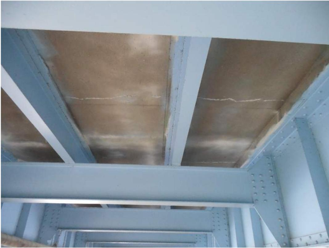
Transverse cracking with efflorescence on bottom of deck
