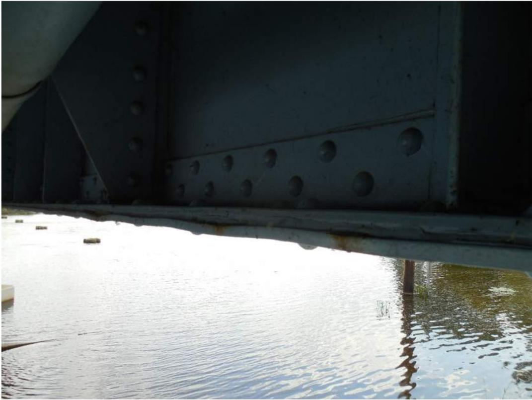
Minor paint failures on bottom flange of girder
