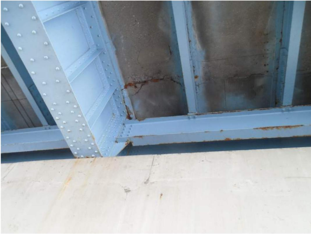
Spalling with exposed steel on bottom of deck
