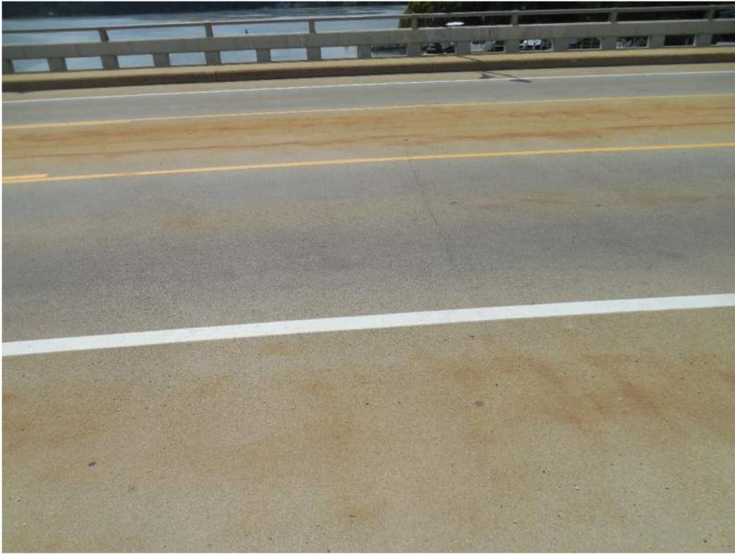
Reflective transverse cracking in epoxy overlay
