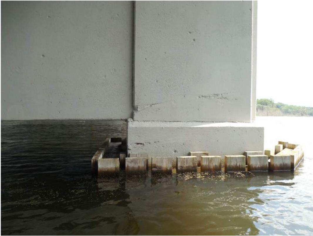
Timber fender nearly submerged
