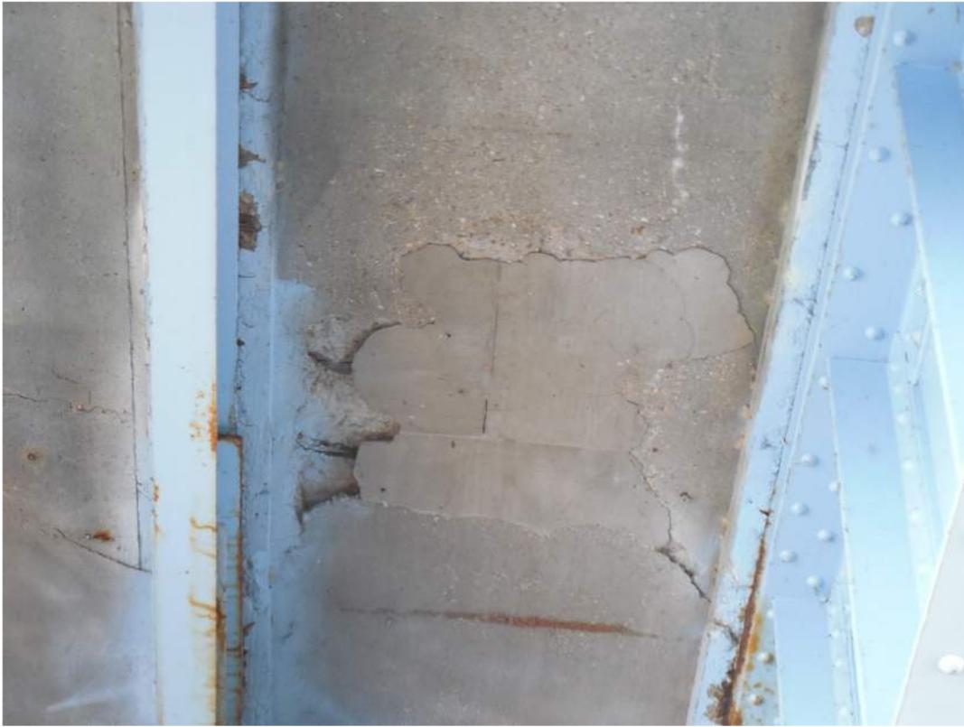
Delamination and spalling on bottom of deck
