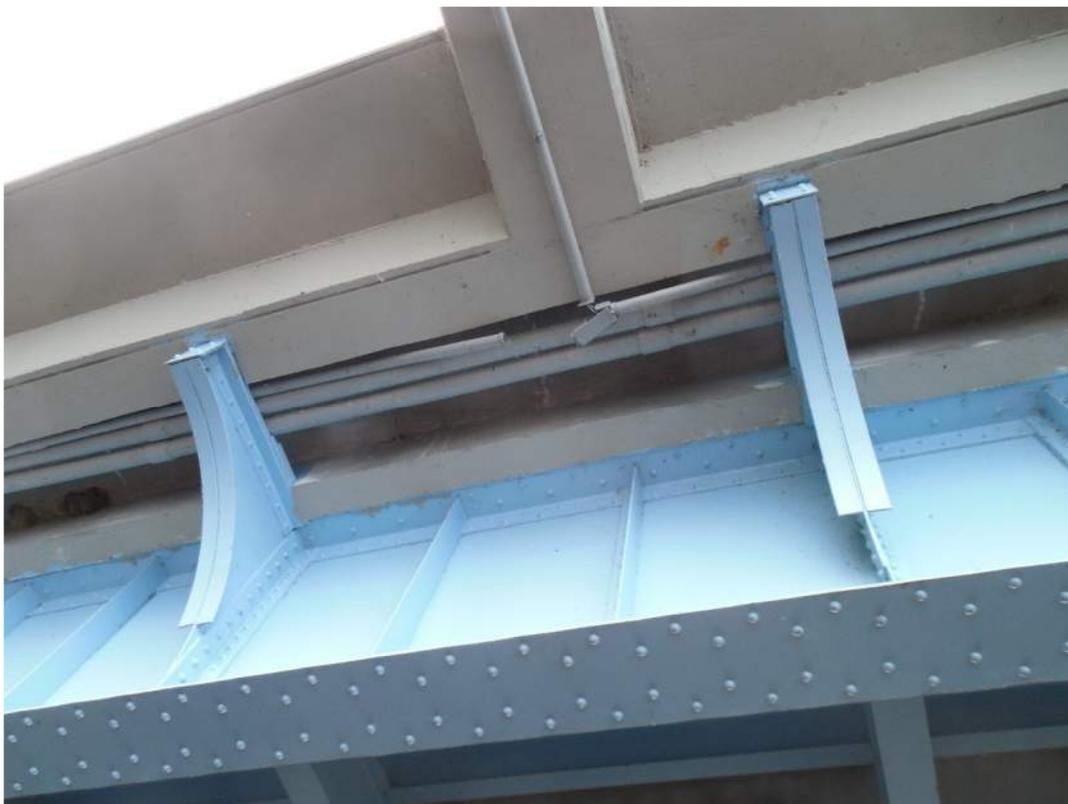
Joint separation in conduit at light junction
