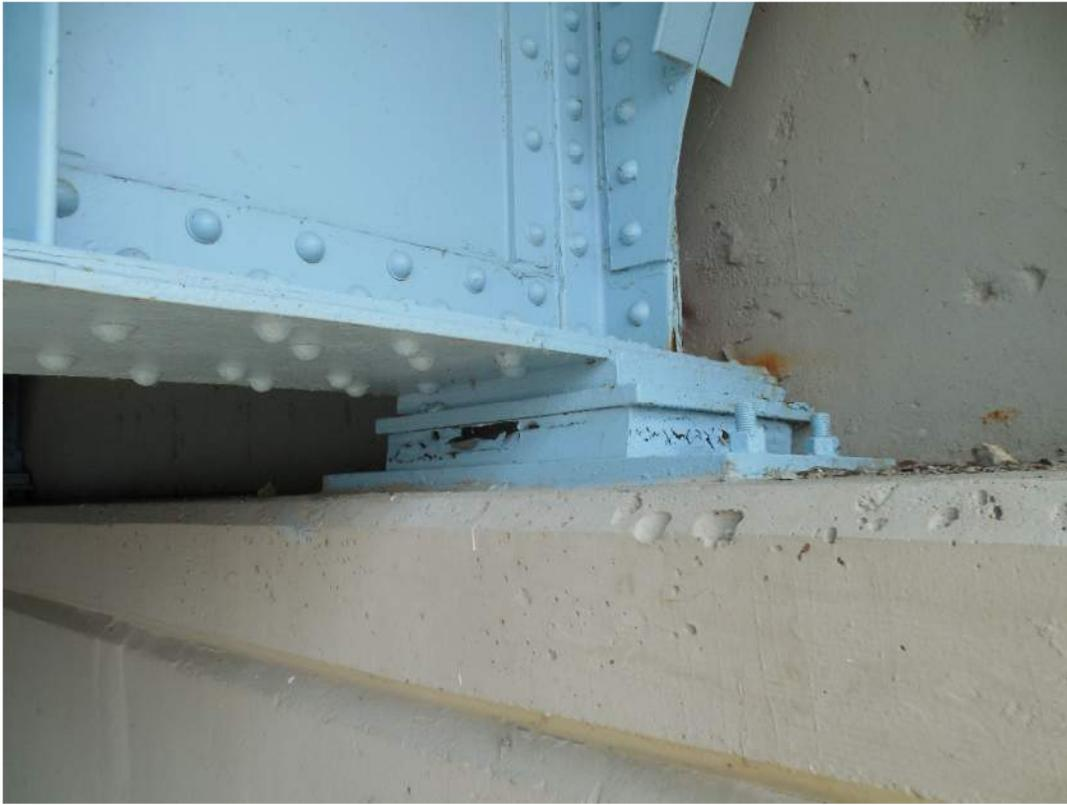
Paint tearing on bearing pad due to movement
