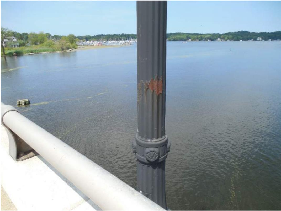
Paint failure and corrosion on light pole
