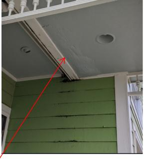
SOFFIT ROTTED AND SIDING WATER DAMAGE DUE TO POOR DRAINAGE OFF OF ROOF(MASON ST AT ADDITION)
