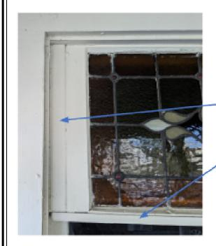
Added pieces of wood to make it fit. The bottom rail of this window should be 1.25" or more. This has a ¾" piece added with a butt joint in the corner. No mortise and tenon which tells me some one manipulated the sash to make it fire into an opening where it doesn't belong.
